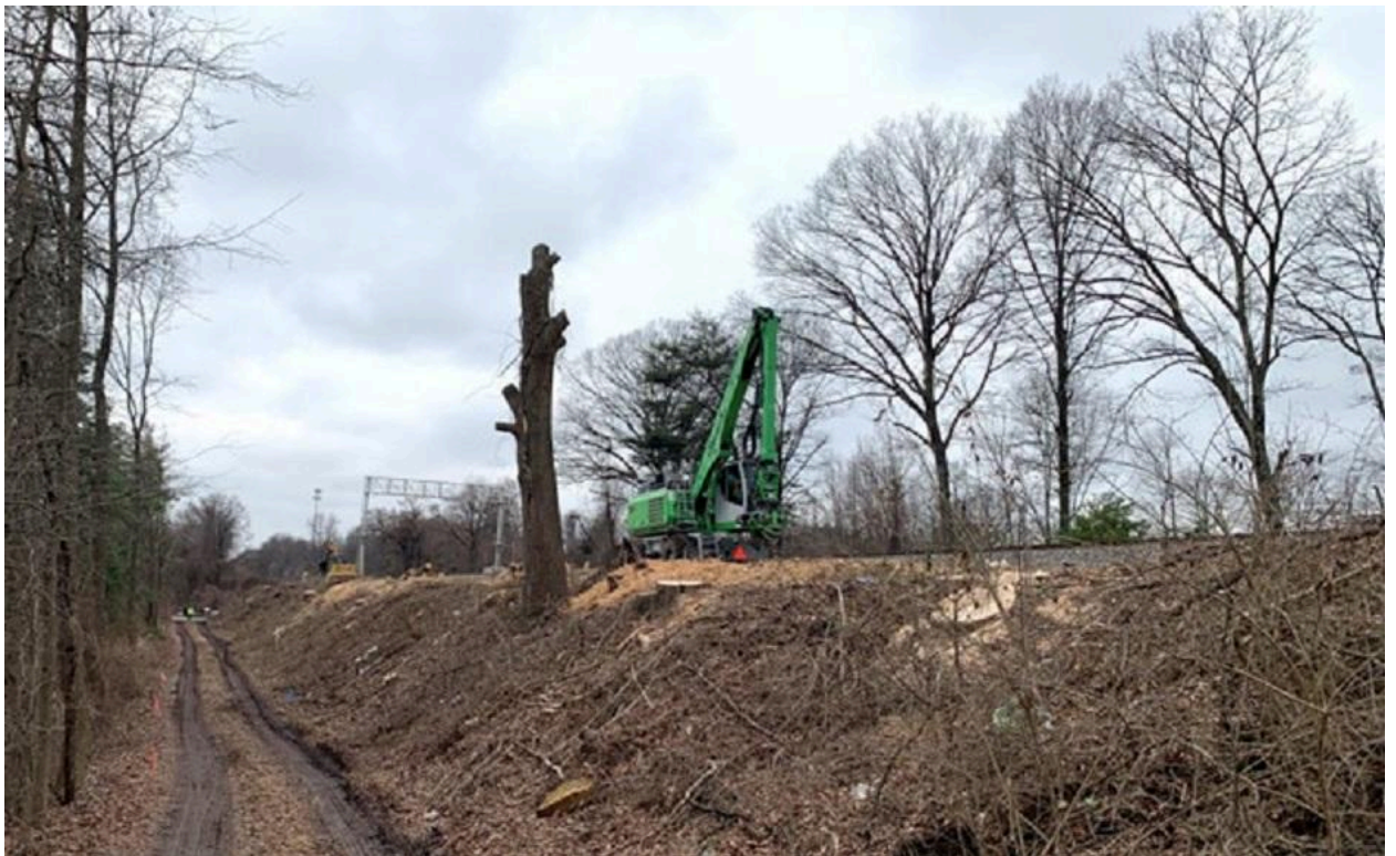
Tree clearing underway for the Franconia to Lorton Third Track
